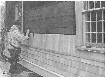
Window frames have been repaired, sills replaced, old electrical systems removed, and reshingling is progressing around the Handy House.
