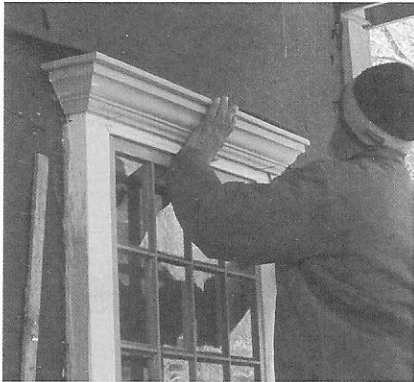
Window frames have been repaired, sills replaced, old electrical systems removed, and reshingling is progressing around the Handy House.
